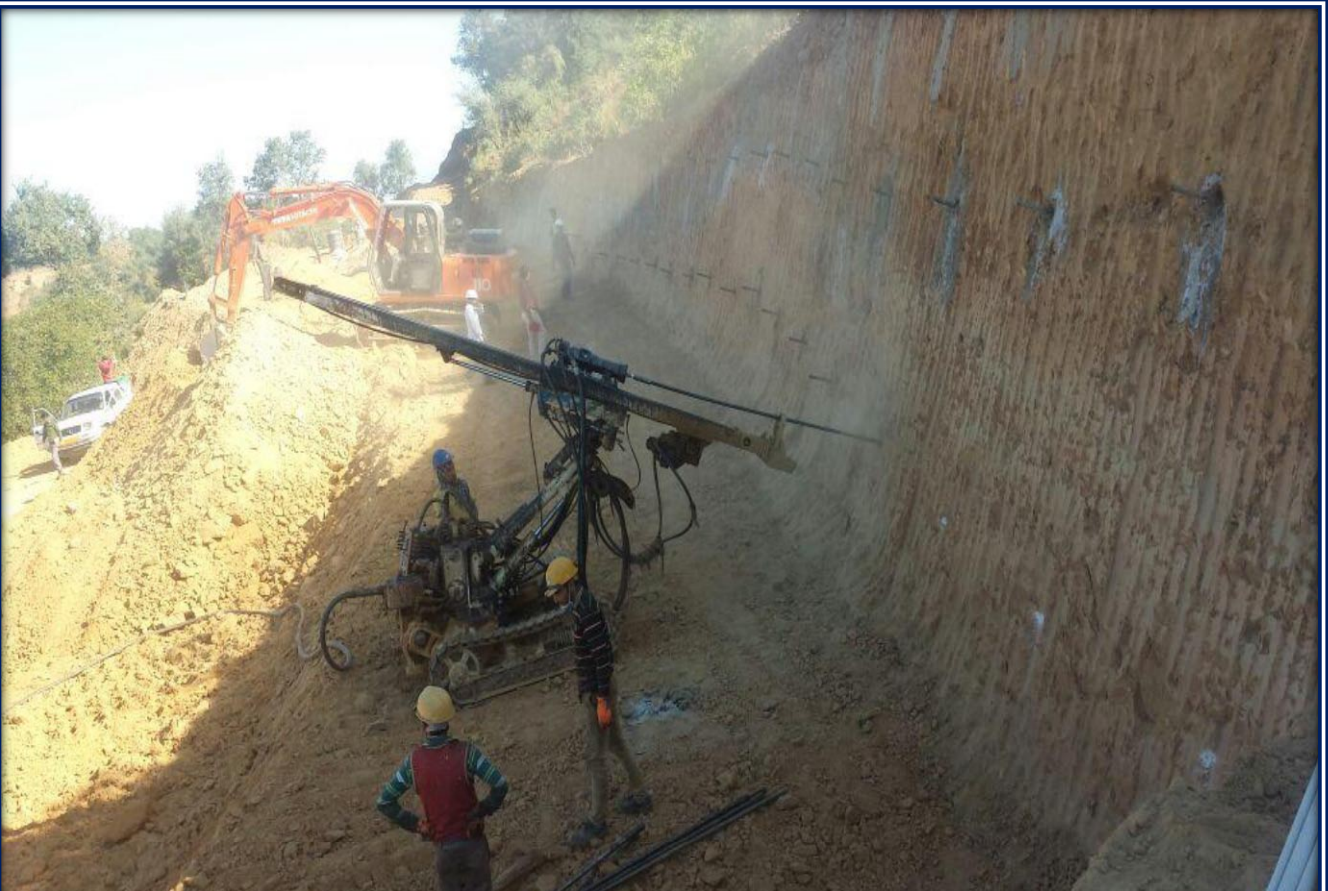
Cut slope protection works through soil nailing technique in progress at CUJ, Jammu
