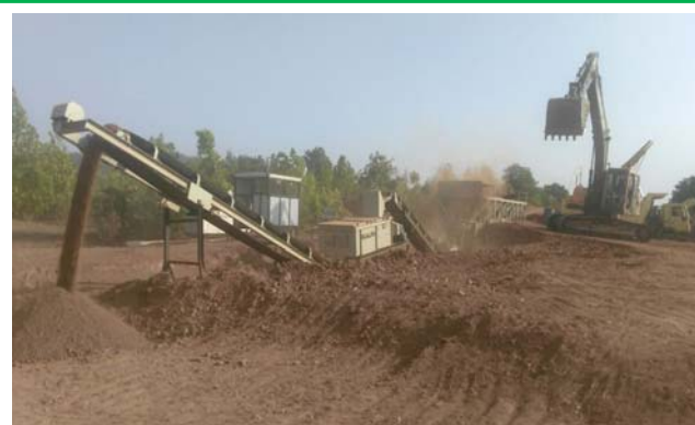
Blanketing Production work of Kharshia work in Progress
