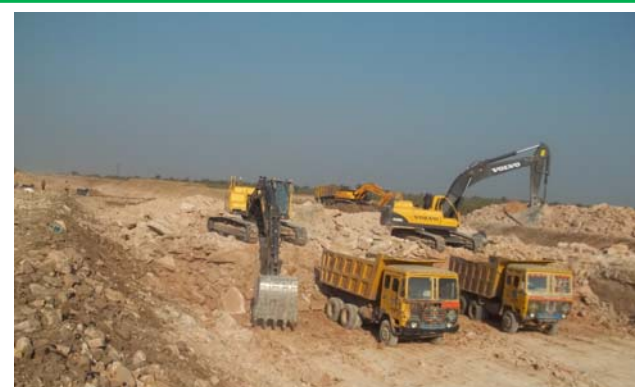
Excavation of Morbi Branch Canal works in Progress
