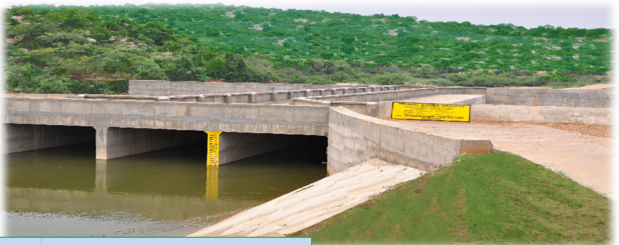
Trough Aqueduct B.T.U.T of SSG Canal (TGP)
