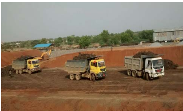
IFFC Project MidManair Karimnagar work in Progress
