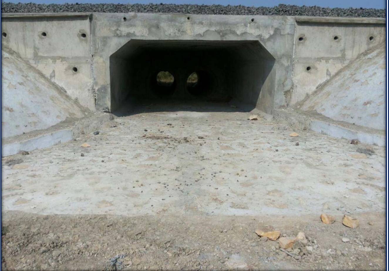
Earthwork in formation, Blanketing, Trolley Refuge and Minor Bridges from Viramgam to Sadla of Viramgam - Samakhiyali Project , Western Railway, Gujrat.
