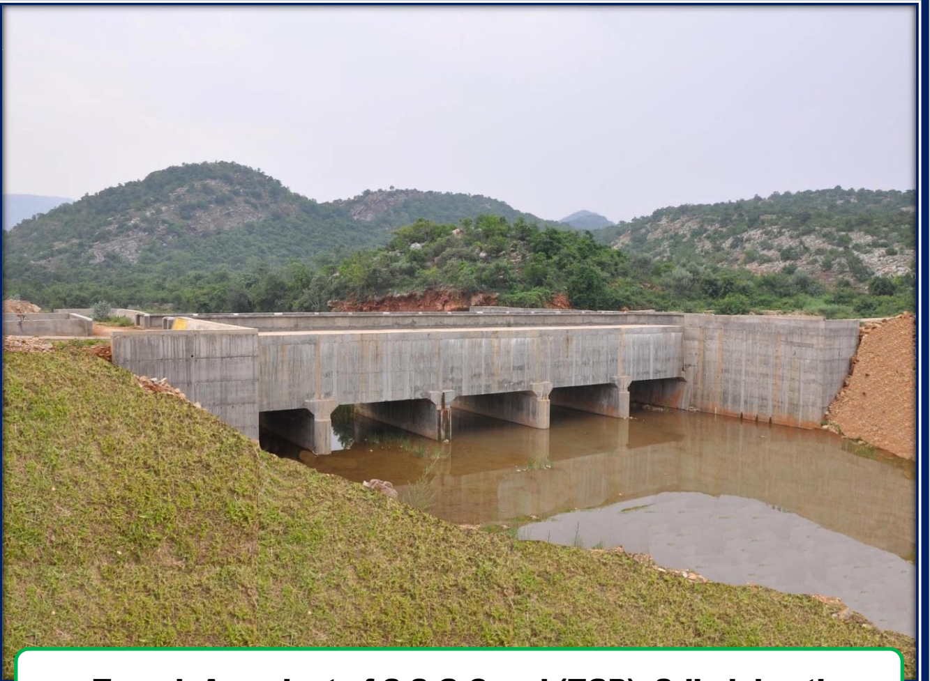
Trough Aqueduct of S.S.G Canal (TGP), Srikalahasti
